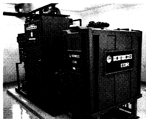
写真1 EDR(宮原簡易水道) Photo.1 EDR system of Miyahara water purification plant
