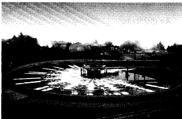
写真3 PABIO Flex 設置例 (2) Photo.3 Example of installation of PABIO Flex (2)
