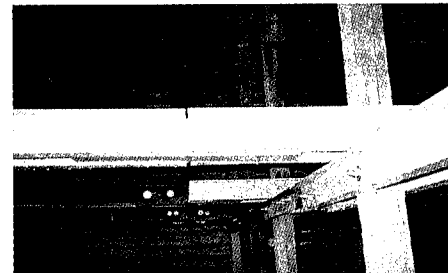
写真6 主構造材(梁) Photo 6 Main structure (Girt)
