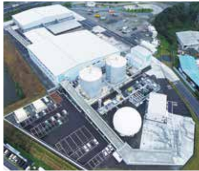
Methane Fermentation Process Facility
