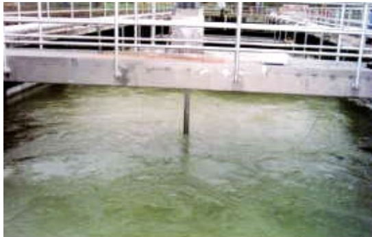
During denitrification operation (mixing)
