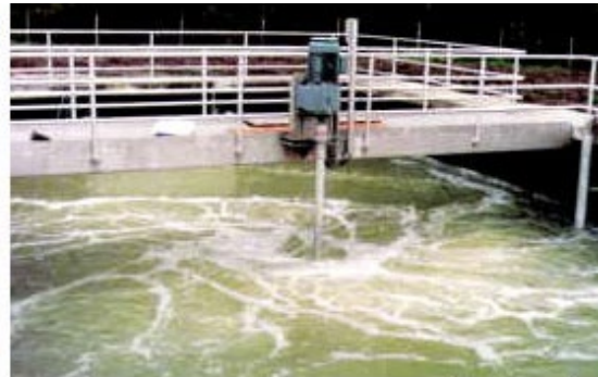
During nitrification operation (aeration)
