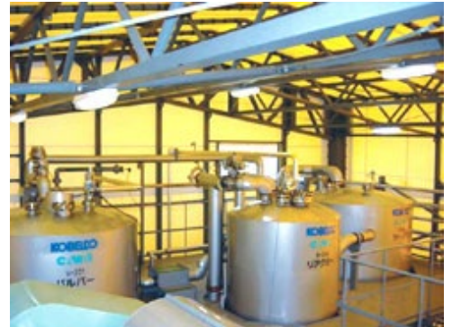
In March 2005, construction technique assessment certificate for sludge solubilization equipment was acquired.
